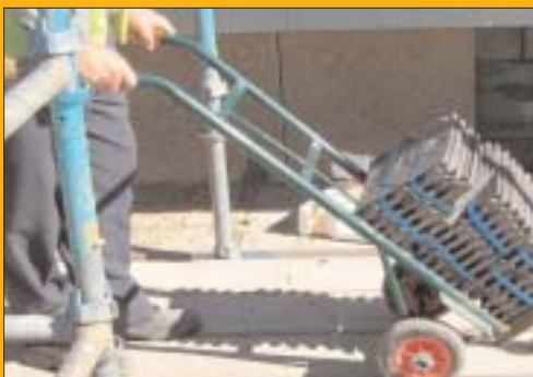
Figure 4 A sack truck being used for moving slates
