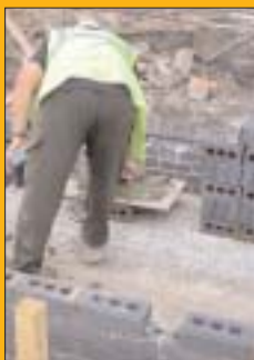
Figure 1 Bending to access mortar and lay bricks at ground level
