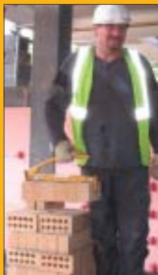
Figure 5 The pincer grip action uses gravity to press the outer bricks together, with no manual force required
