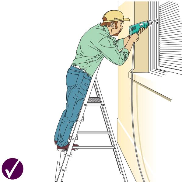
Figure 3a Correct - rungs facing work activity
