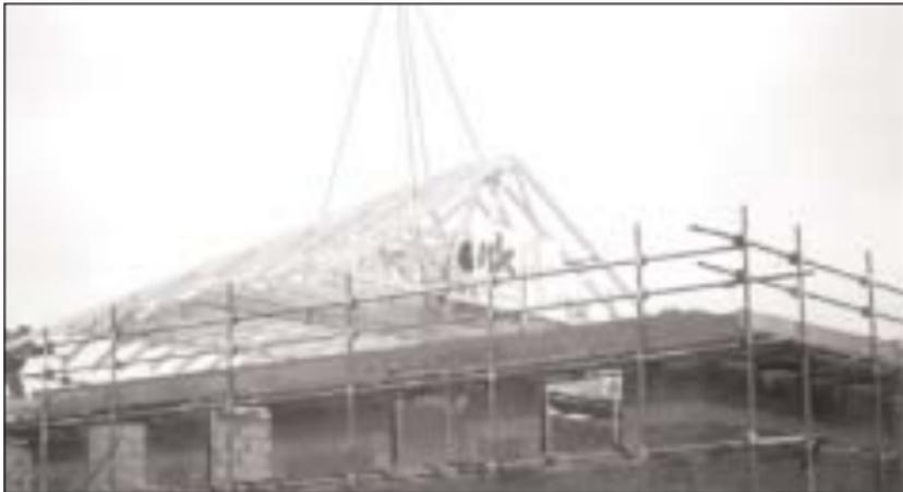
*Roof truss built on ground and lifted into position avoiding the need to work over open joisting later on*
