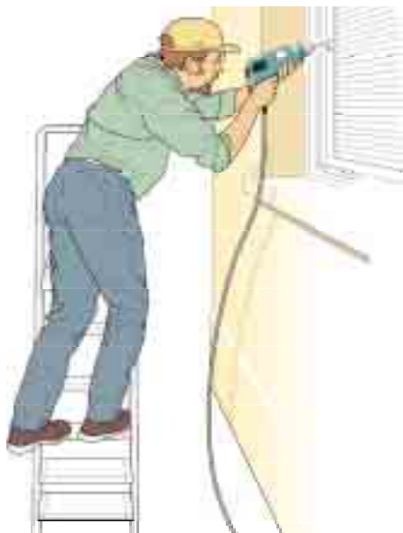
Figure 2a Incorrect - steps side-on to work activity
