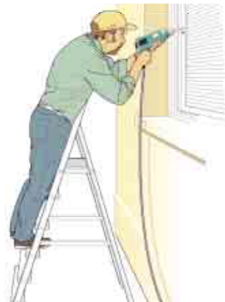
Figure 2b Correct - steps facing work activity
