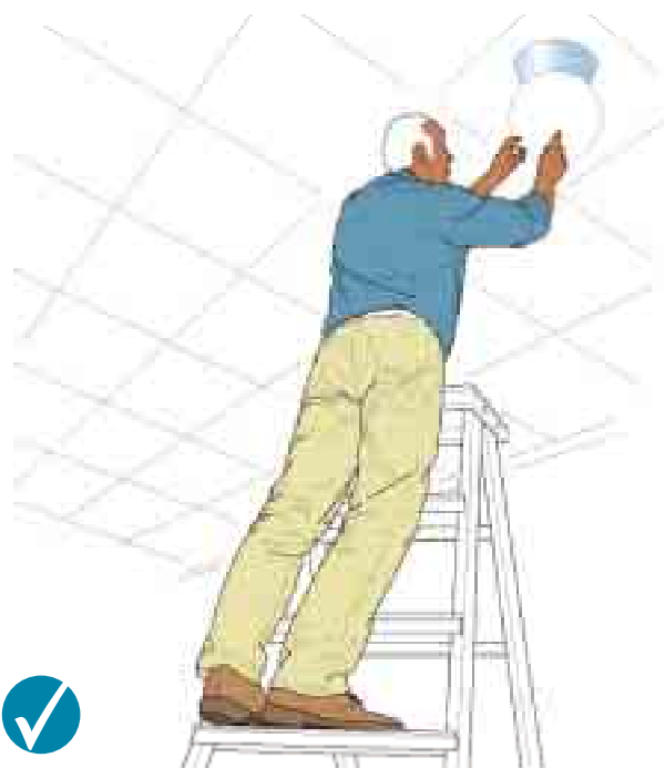
Figure 12 Correct - three clear steps. Don't work any higher up this type of stepladder
